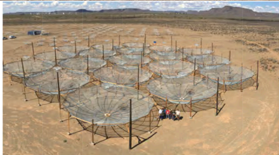
Fig. 1.— Rendering of the 320-element core (left) of the full HERA-350 array and picture of 19 HERA 14-m, zenith-pointing dishes (with PAPER elements in the background) currently deployed in South Africa (right).
